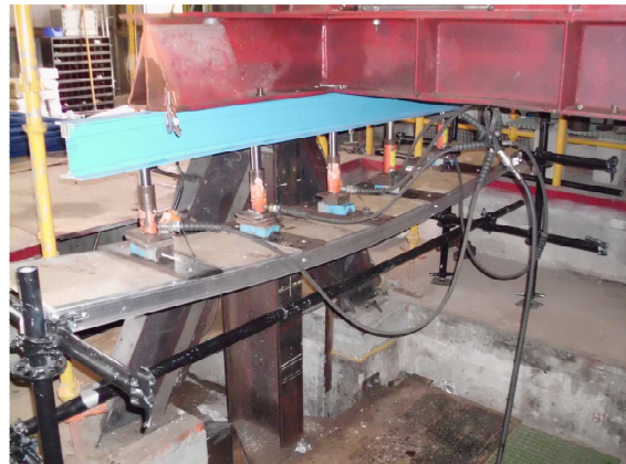
Typical failure by deflection
